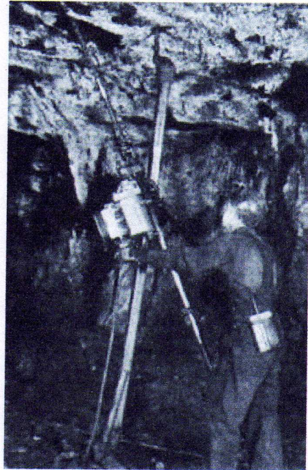
Preparing for blasting with the use of a compressed-air drill
